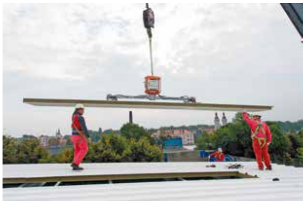
Pic. 8 and 9. Assembly of roof panels.
